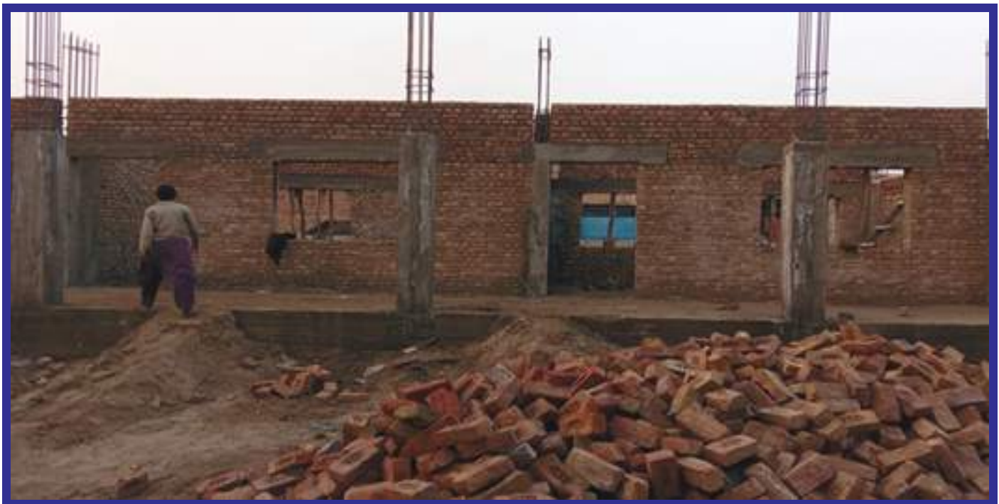
Additional Classrooms under Construction (GBELS-ATUR JHOKIO SEMIS CODE-417020380)
